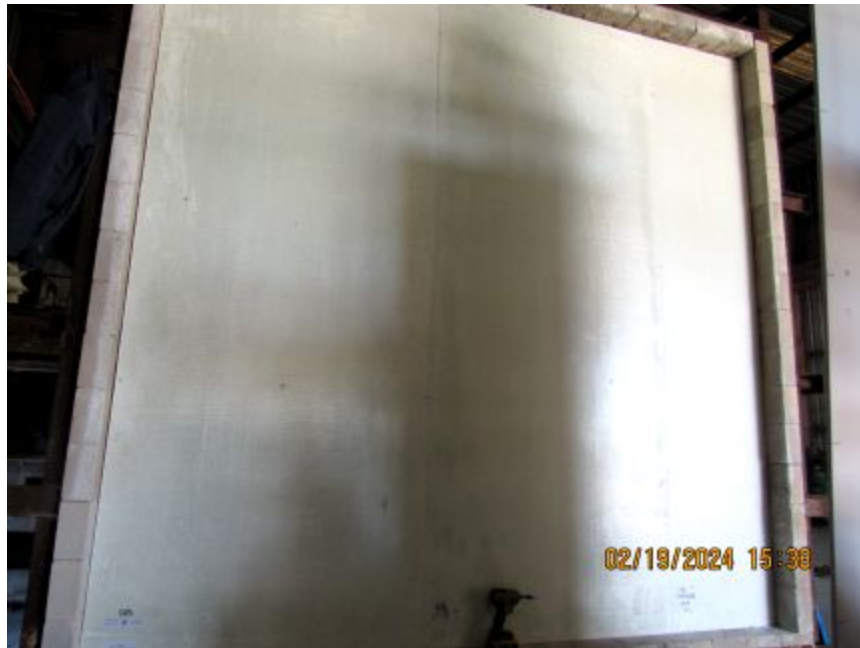
Photo No. 20 Armor Core Panels Fastened into Gypsum
