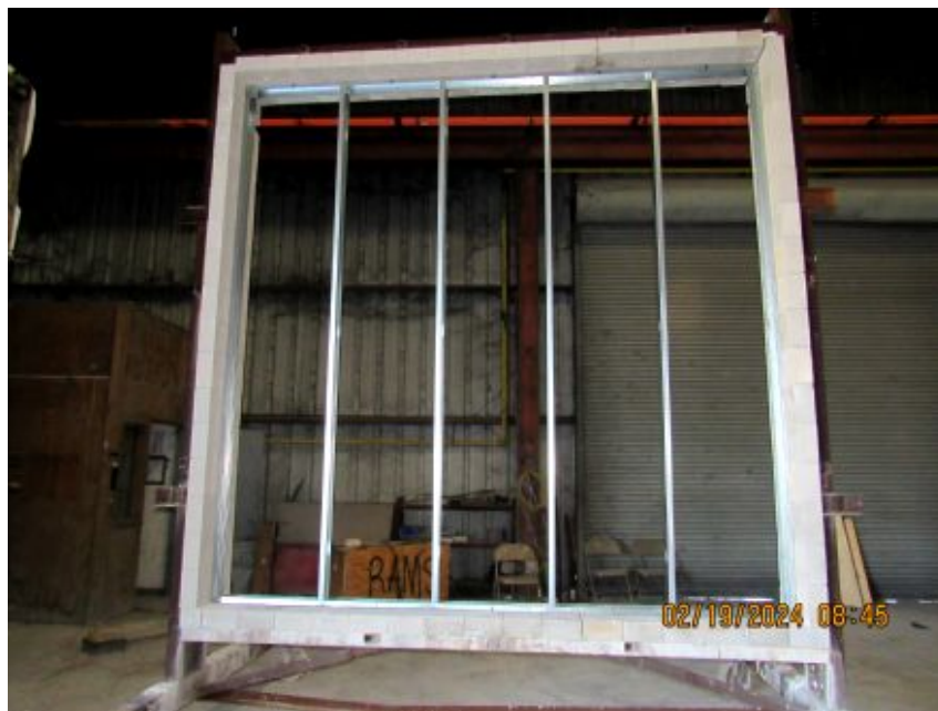
Photo No. 2 Studs and tracks installed into frame
