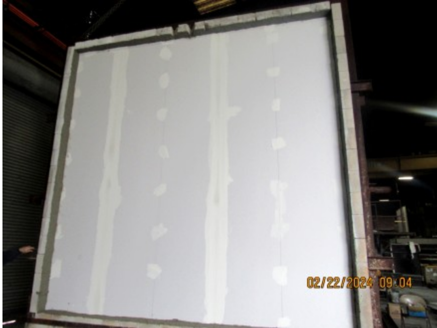
Photo No. 3 View of Completed exposed side
