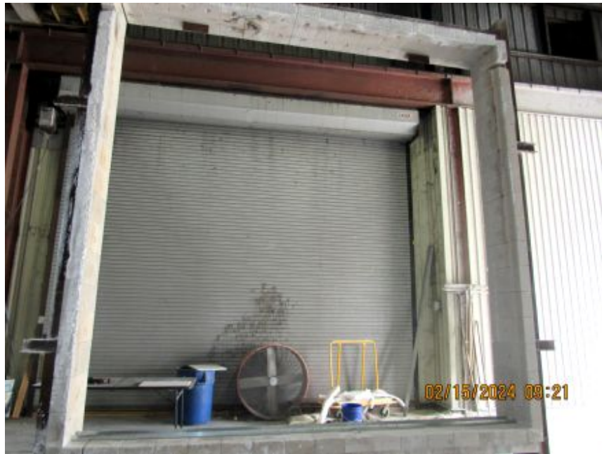
Photo No 1. View of Test frame before Installation
