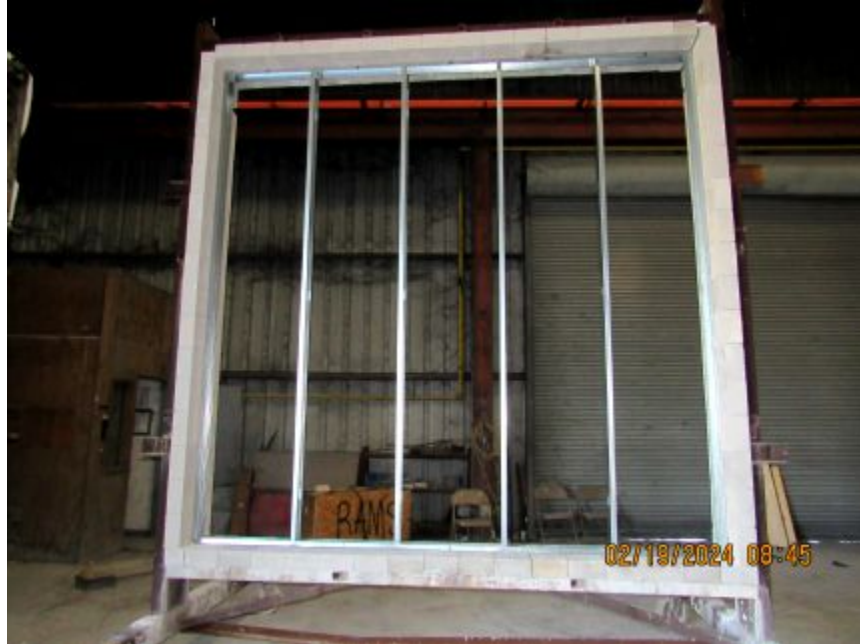
Photo No. 17 Tracks and Studs Installed Into Frame
